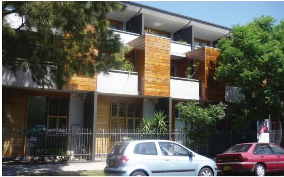
Figure 5.xx Example of developments that use a range of building materials, Alexandria
